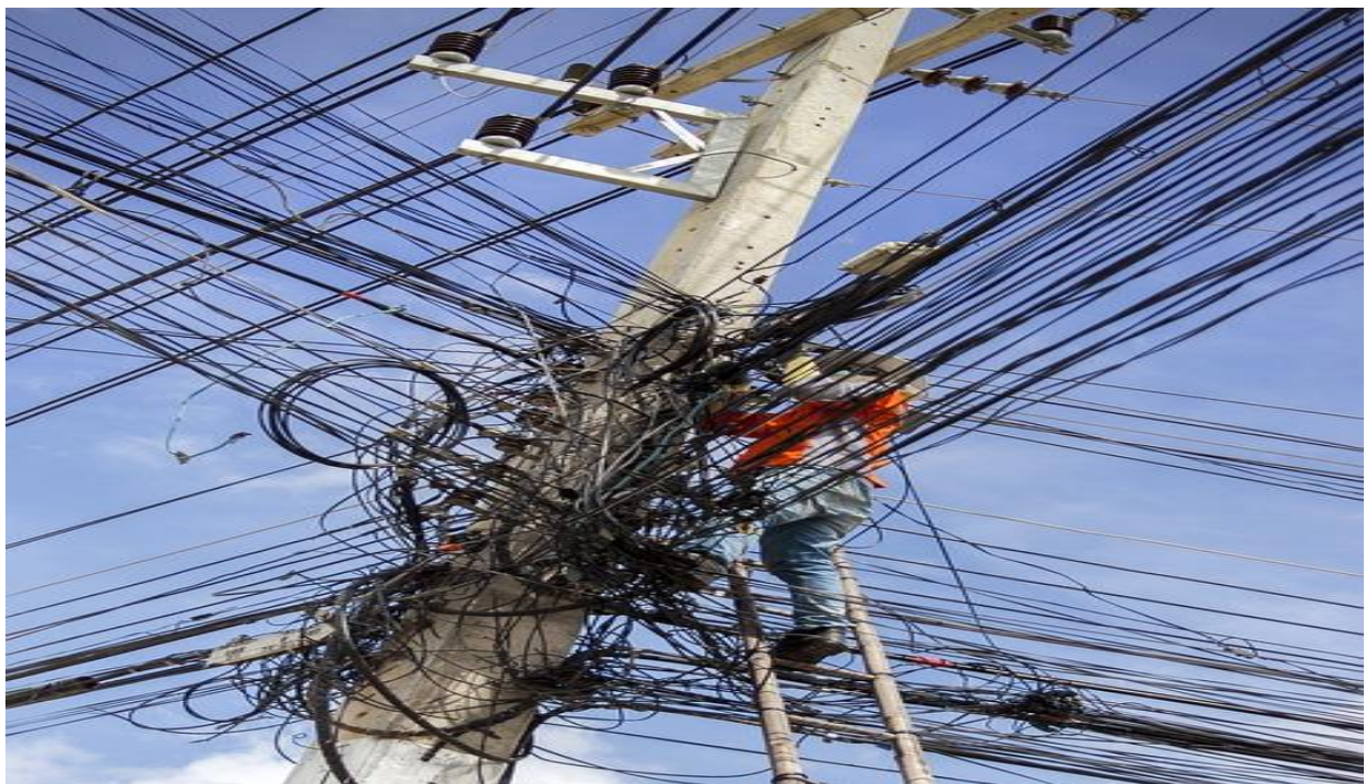
Figure 12: Representative old telephone network having drop wires as last mile connectivity
